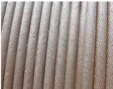
Cables affected by pitting caused by Hydrogen Sulfide.
